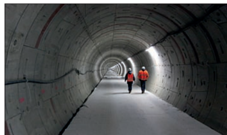
The European XFEL tunnel construction, which began in July 2010, is now complete. (Image credit: European XFEL.)
